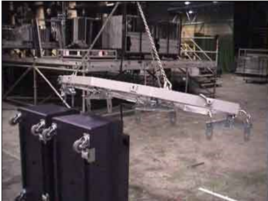
Fig 4.5-6 Enclosures aligned near the grid
