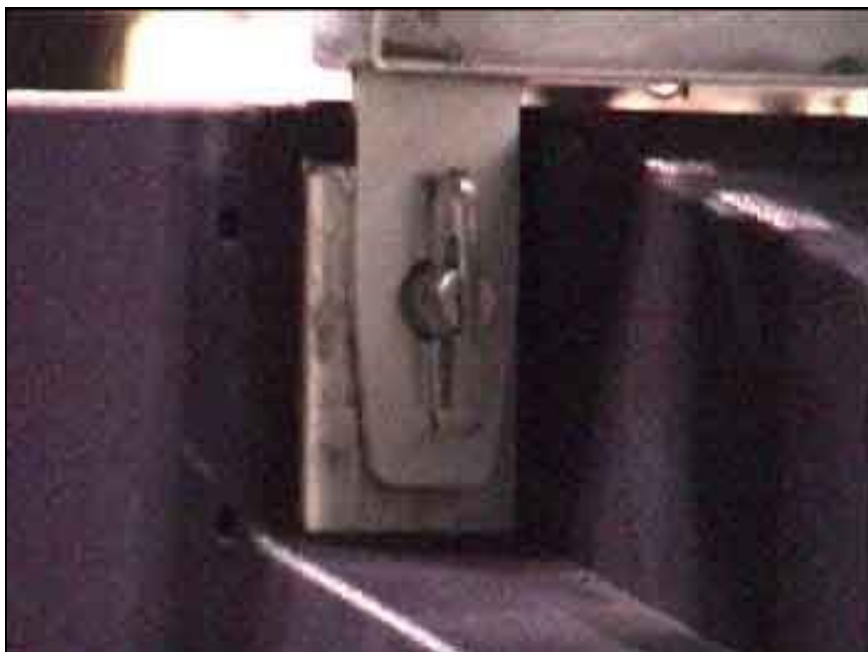
Fig 4.5-10 The toggle pin mated with CH5 column hanger - and repeated with each enclosure on the top row.
